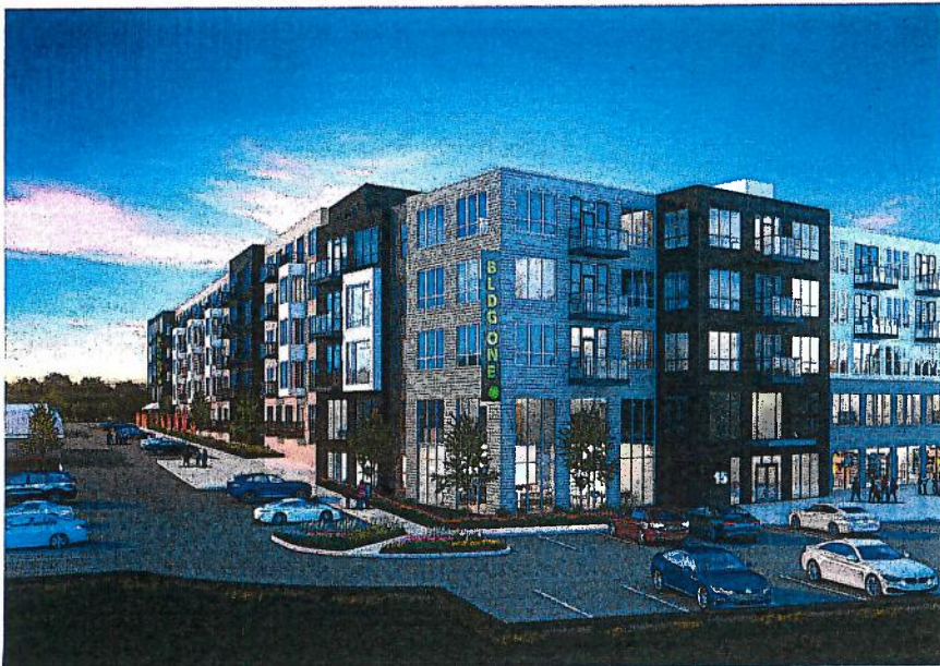
Southwest From Entry Road
