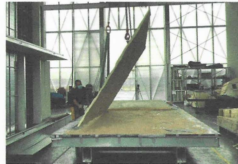
GFRC Facade 28/10/2020, WOHO LAB - WETLAB >>>>
