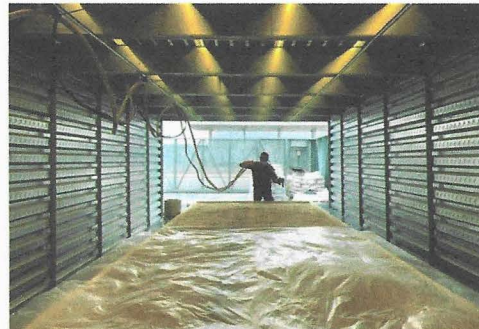
GFRC Facade 28/10/2020, WOHO LAB - WETLAB >>>>
