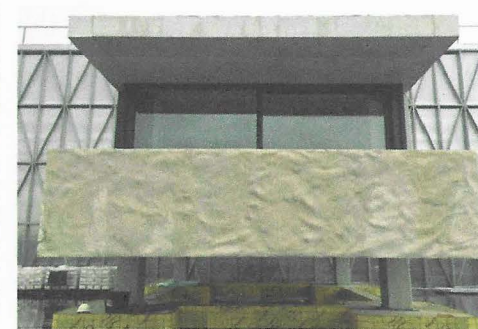
GFRC Facade 28/10/2020, WOHO LAB - WETLAB >>>>
