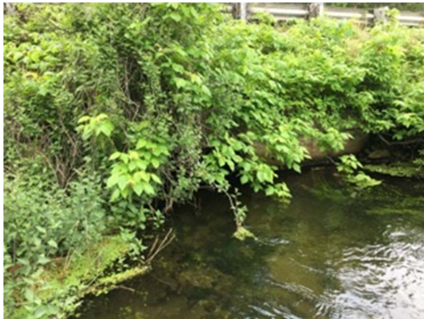
Downstream box culvert (Hager Pond outlet)
