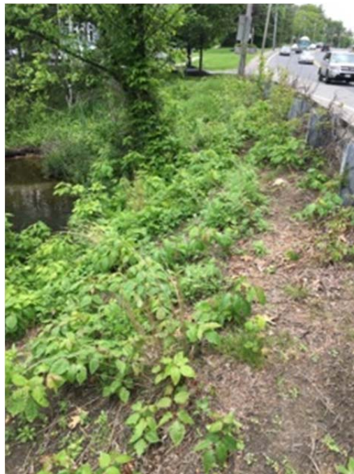
Looking west along Route 20 at culvert crossing outlet to Hager Pond
