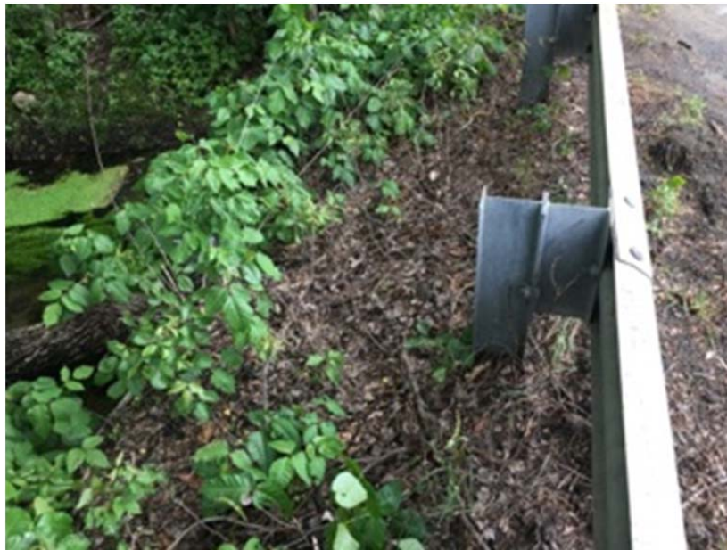
Upstream box culvert – face of guardrail approximately 6' off face of culvert
