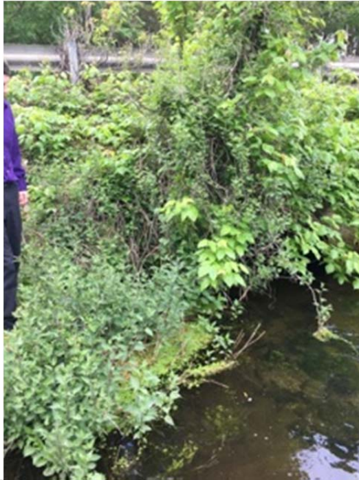
Downstream box culvert (Hager Pond outlet)
