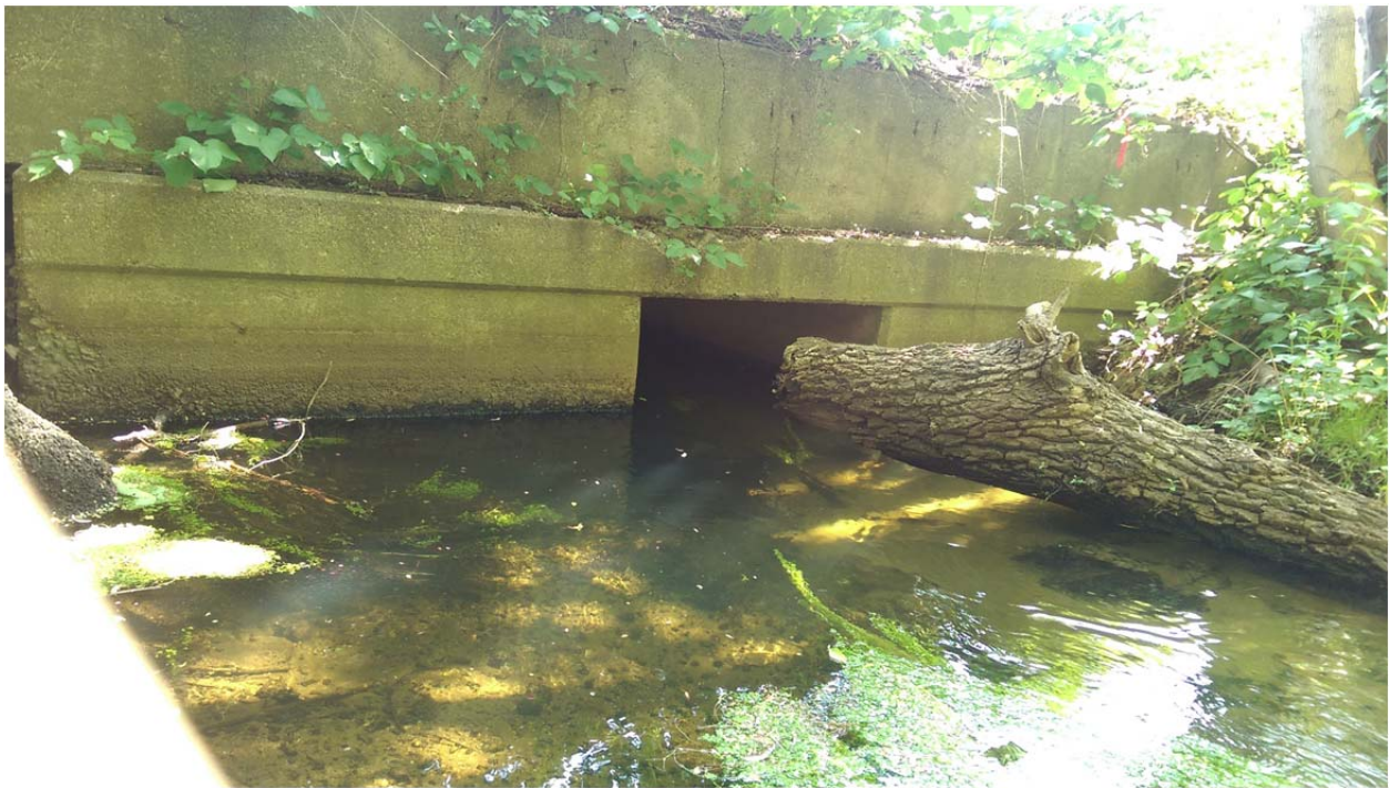
Headwall at upstream (Northern) headwall
