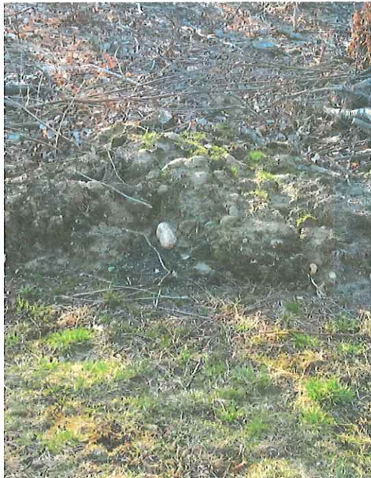
soil and debris from lamp installation in buffer zone
