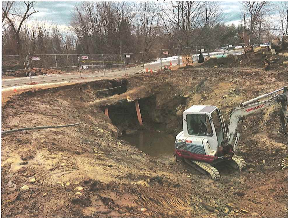
Excavator in hole between inlet and outlet pipe.
