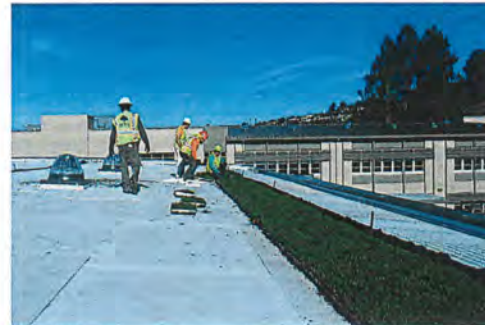
EXAMPLE LIVE ROOF INSTALL PHOTO
