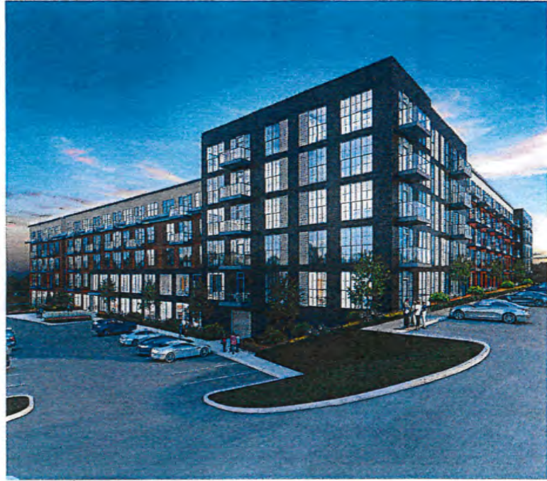
Southeast Corner From Access Road
