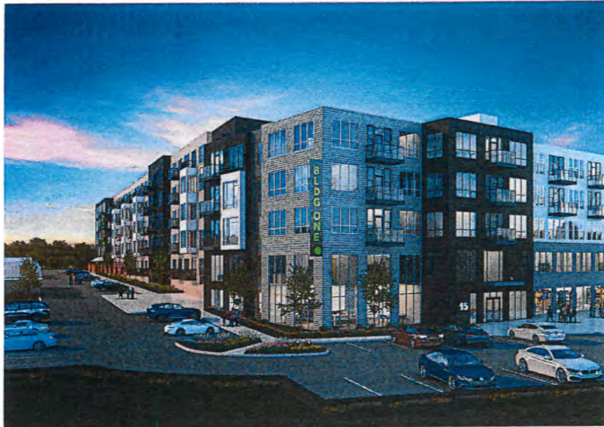
Southwest From Entry Road
