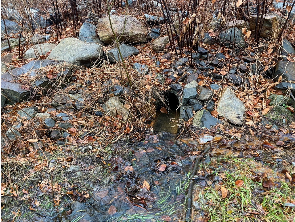
Figure 3 - Flared End Section Outlet
