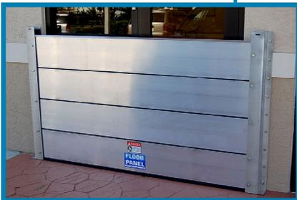
Example of flood shield over door opening
