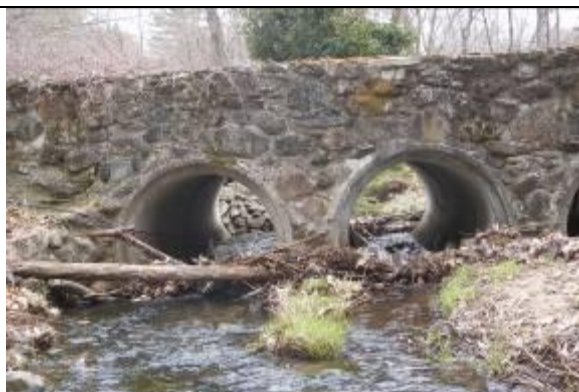
F11 Rock wall bridge driveway w blockage
