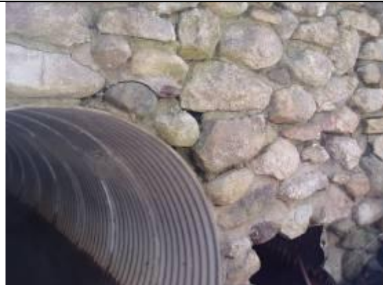
#6 Cracked culvert. Close up of #5 culvert
