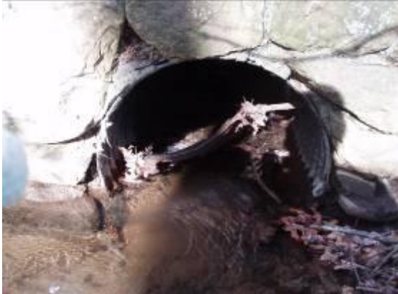
#13 Hemenway Ext Broken SE culvert
