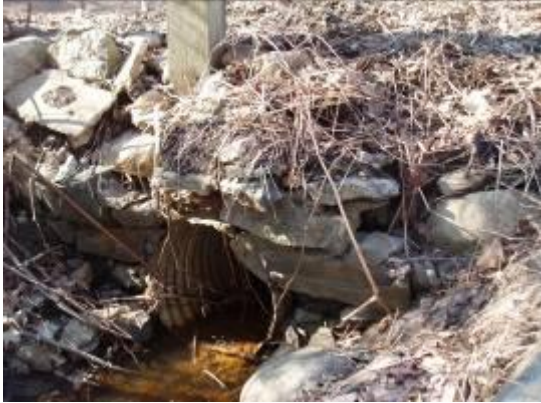
#9 C5? Concord Rd Culvert, rocks ready to fall
