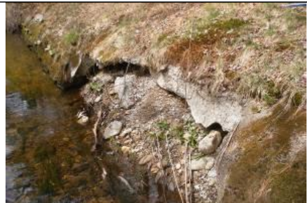
G11 Undercut Channel Breakage
