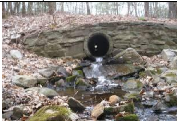
G10 24-inch Drain with Rapid Flow of Water
