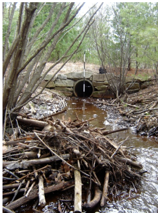
(photo below) other side of culvert (opening) almost completely clogged
